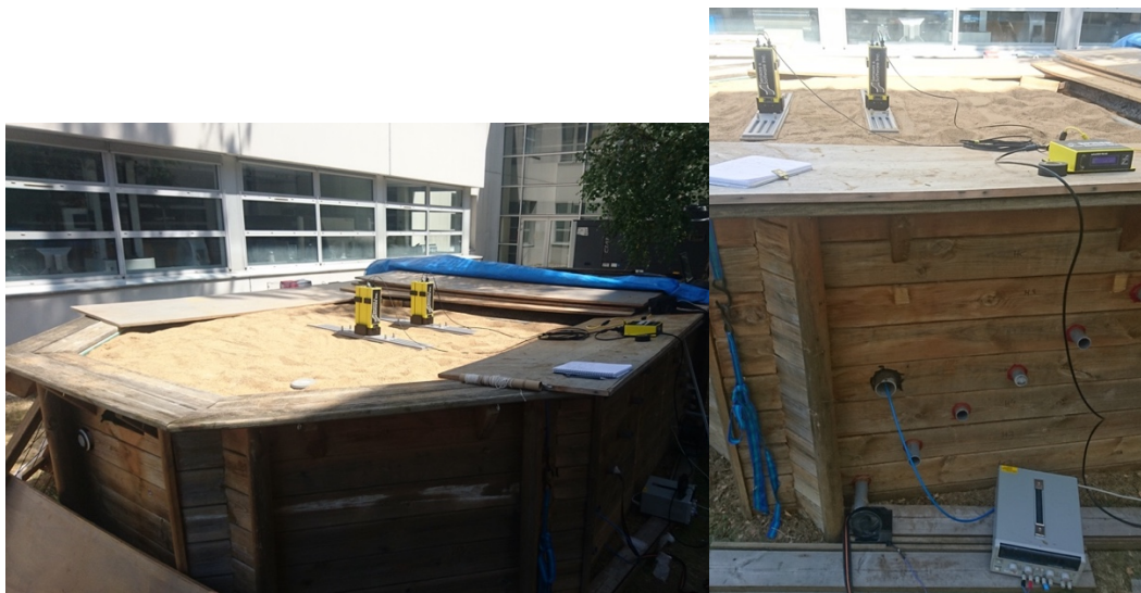
Figure S2. The sand-pit for the demonstration of sub-surface wireless sensing (left). The GPR is over the sand-pit and the sensor is located in a pipe where H 2 S is injected into the pipe as gas phase (right) at different depths (from 0.2 to 1m).
