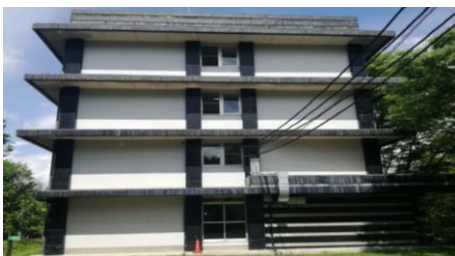
Fig. 9. Experiment with a four-floor building as target.
