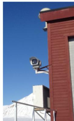
Optical link in Ny-Ålesund (2.45 and 5.8 GHz band use prohibited since reserved for radiotelescope deep space measurements).
